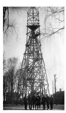
In 1931 for observation purposes a 42 m high triangulation wooden tower was built above the Struve point. For several summers, the teaching staff and students of the University of Latvia conducted astronomical and geodetic research and measurements
