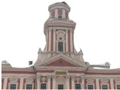
Tower - view from the bottom
